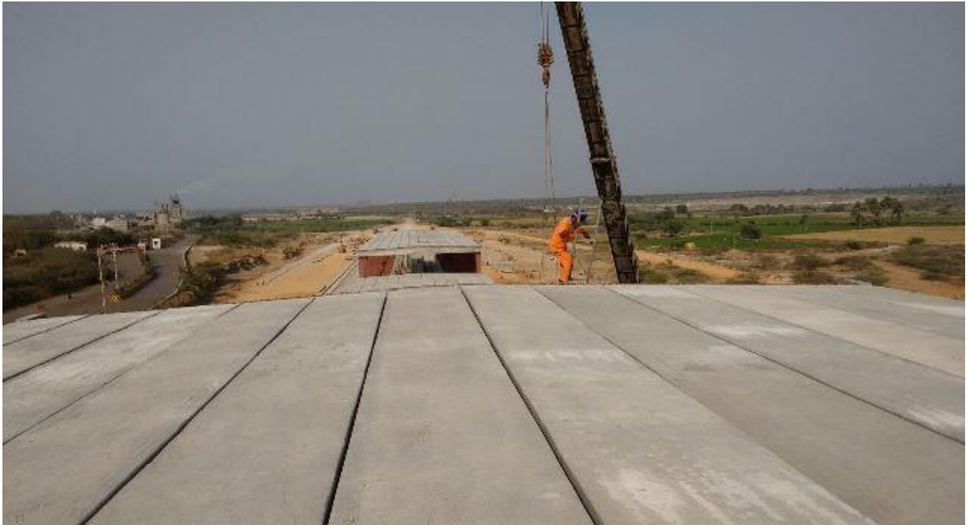
Erection of roof slabs
