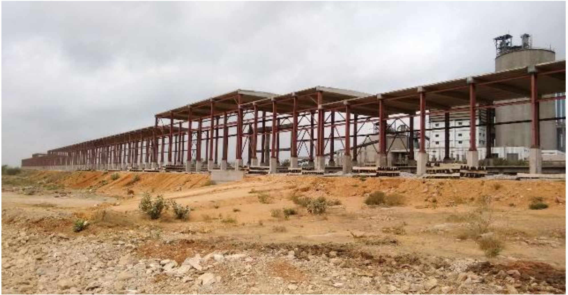
A portion of the 750m long shed
