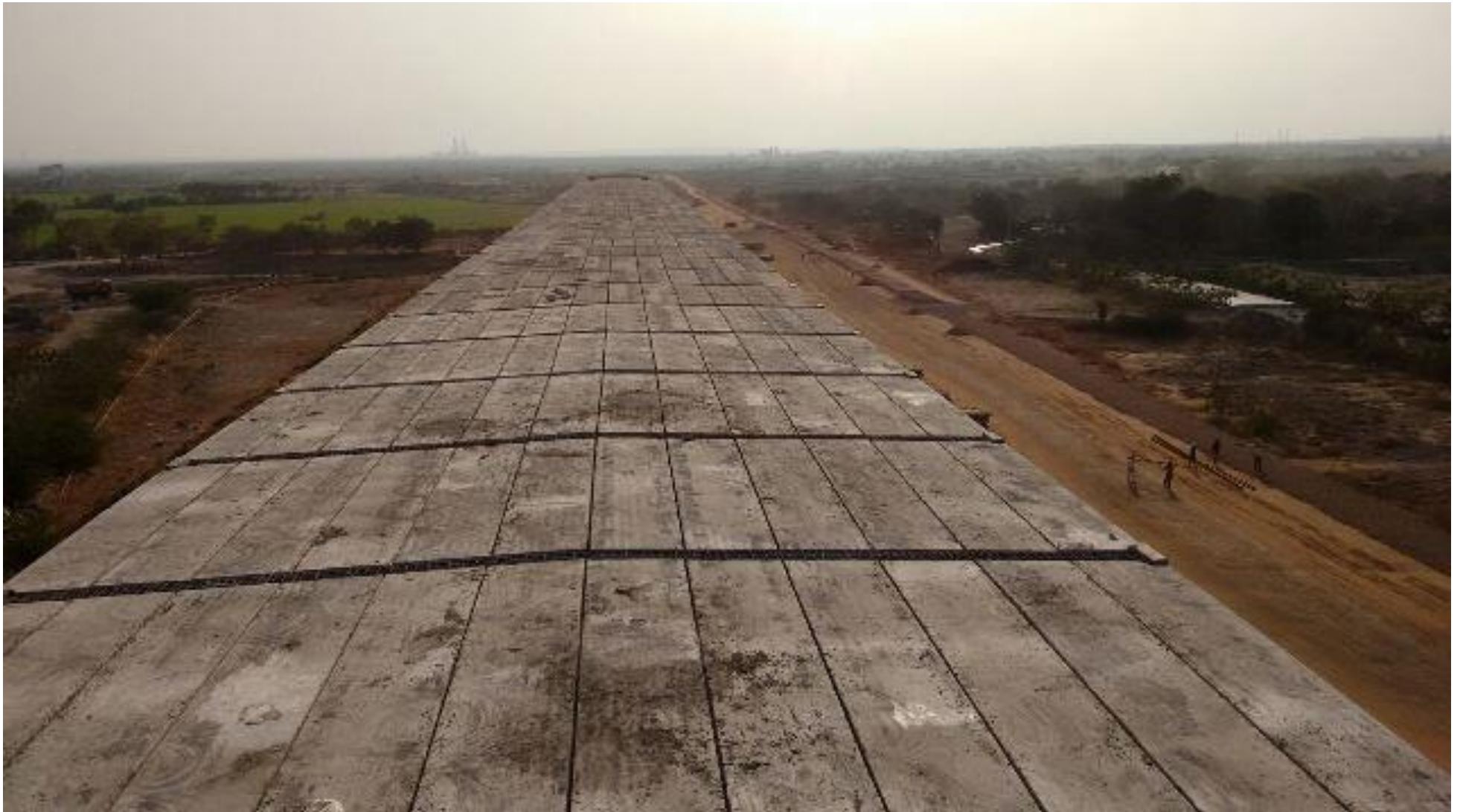
The erected roof slabs
