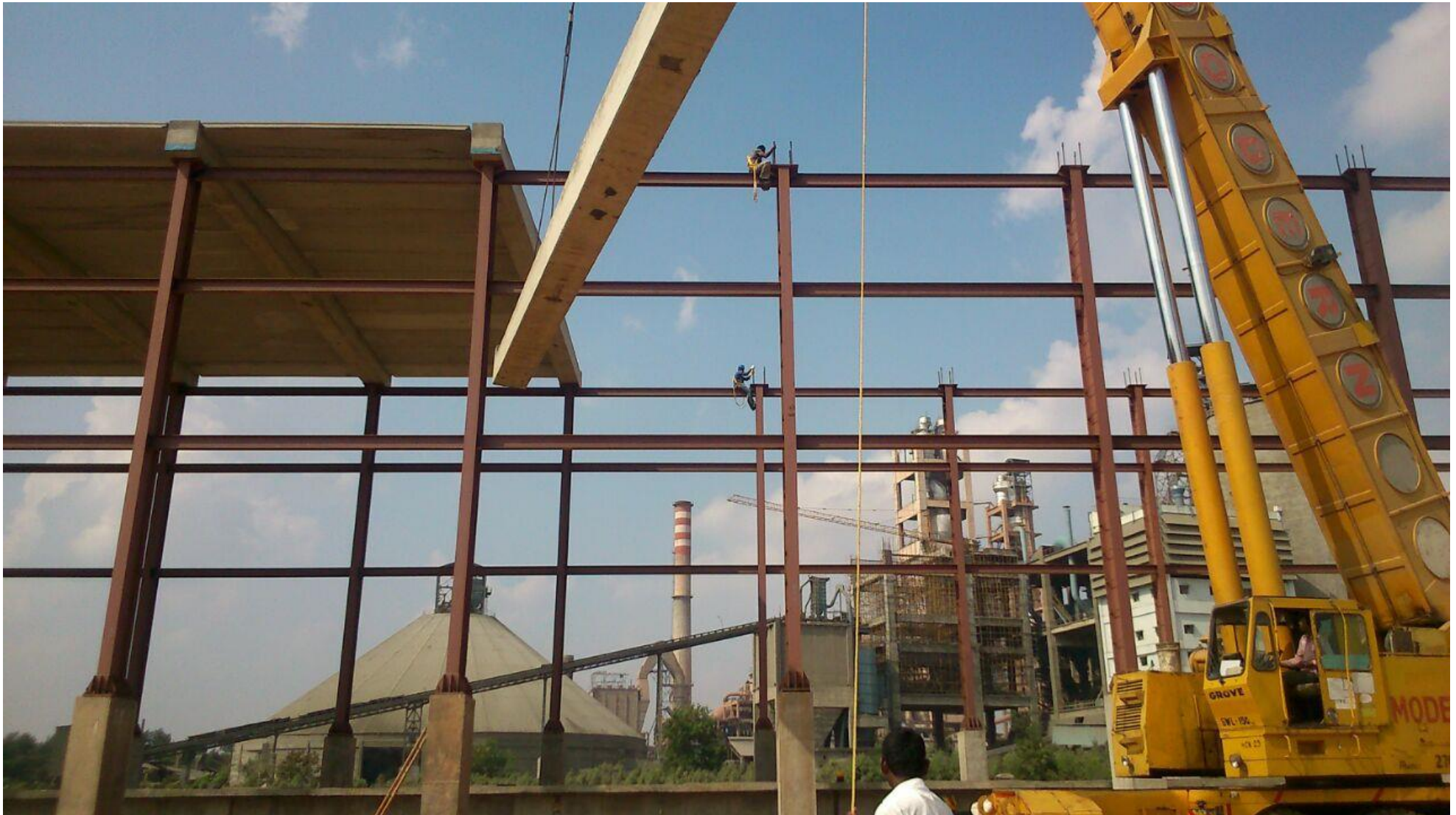
Erection of Rafter elements
