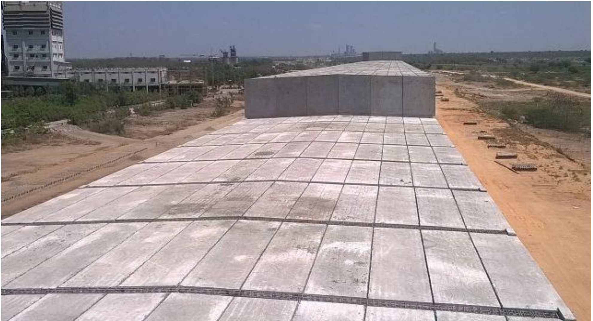
The erected roof slabs
