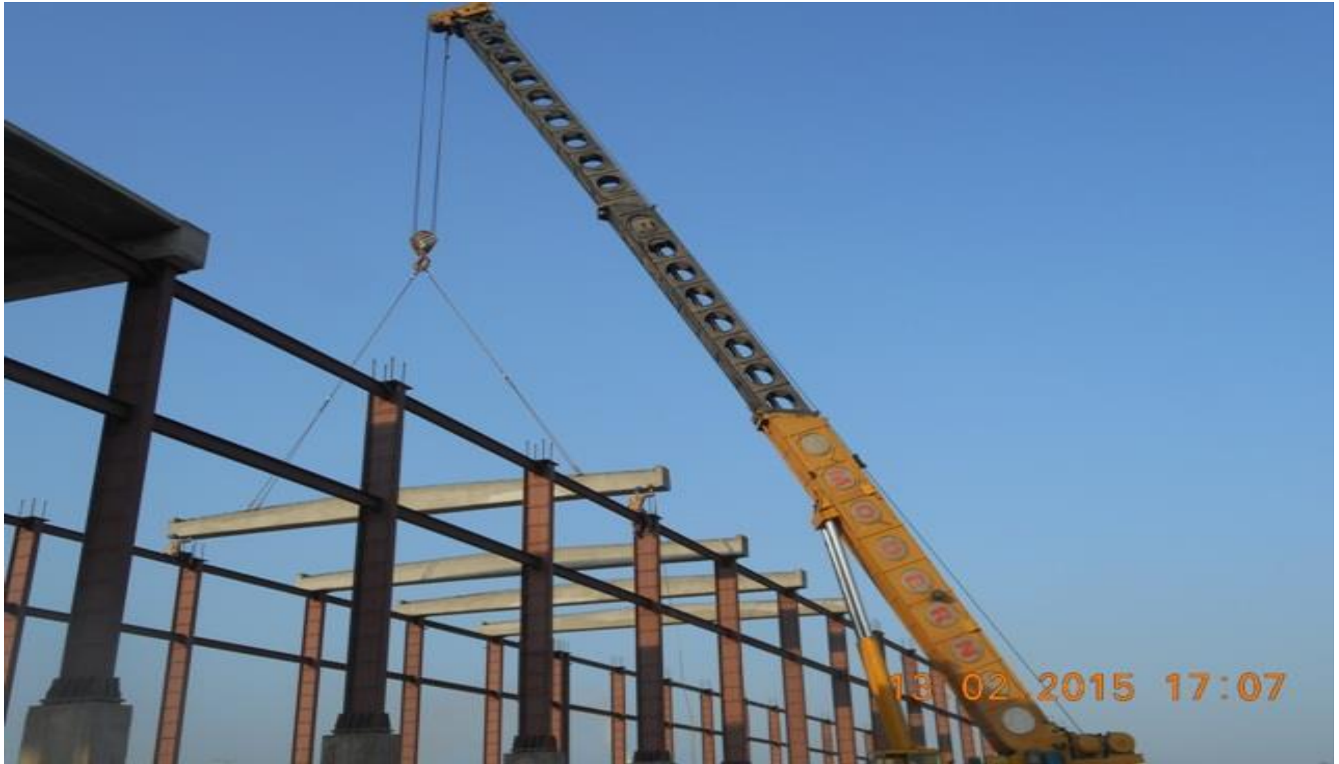
Erection of Rafter beams
