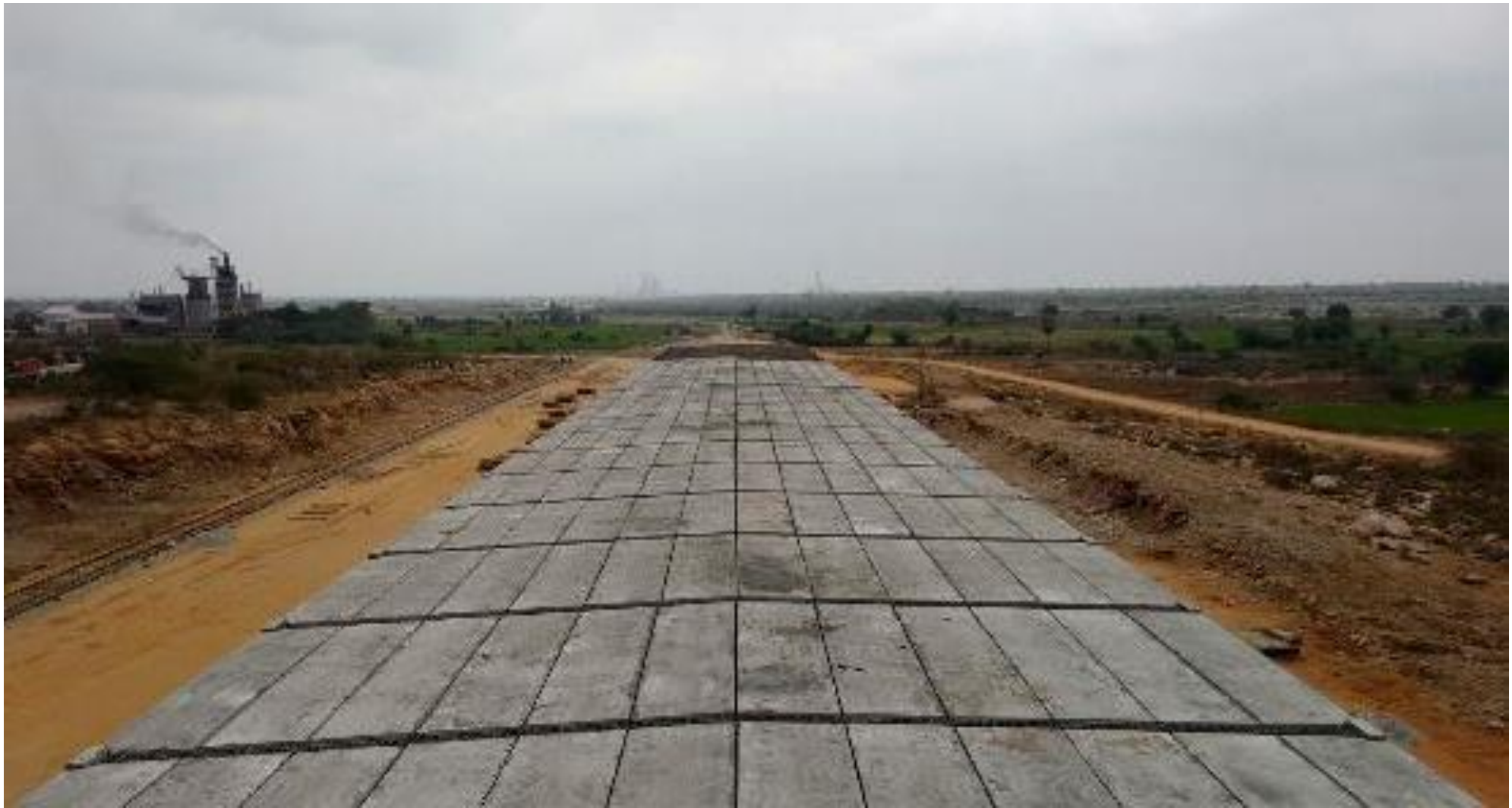
The erected roof slabs
