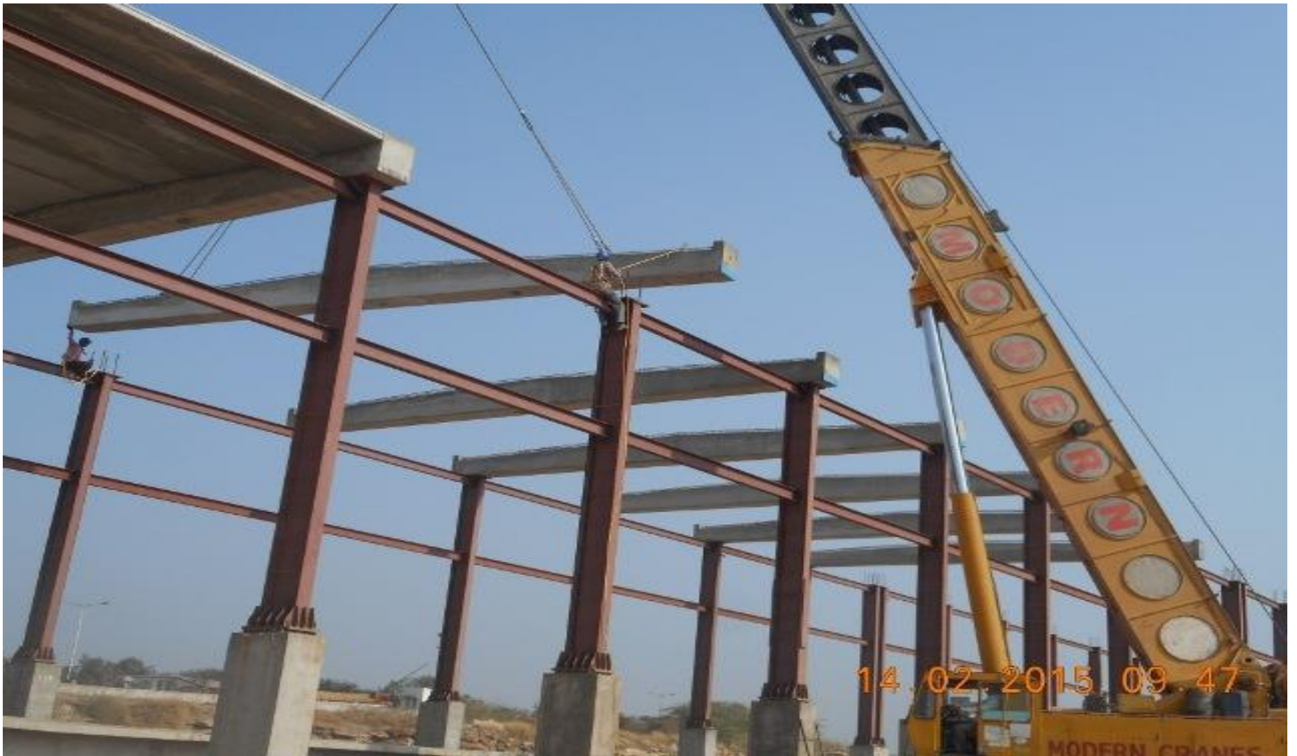
Erection of Rafter elements
