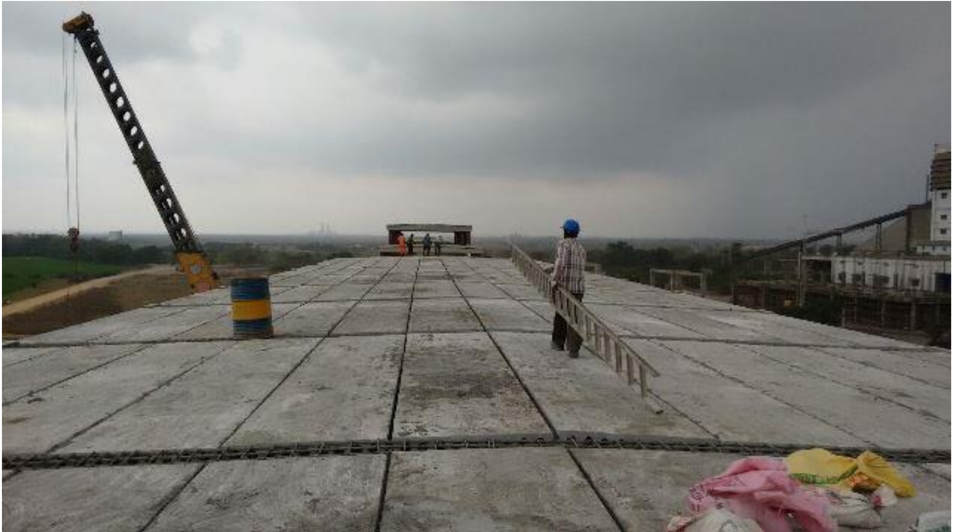
Erection of roof slabs in progress
