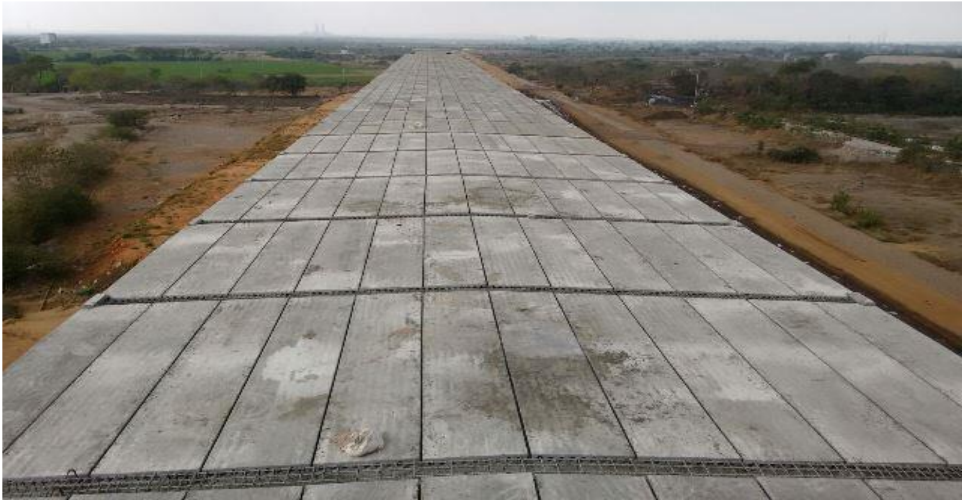
The erected roof slabs
